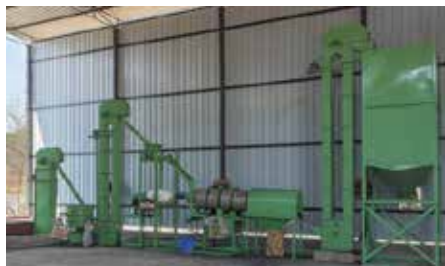
TCTD pilot plant for reclamation, commissioned at Govt. Polytechnic, Kolhapur
